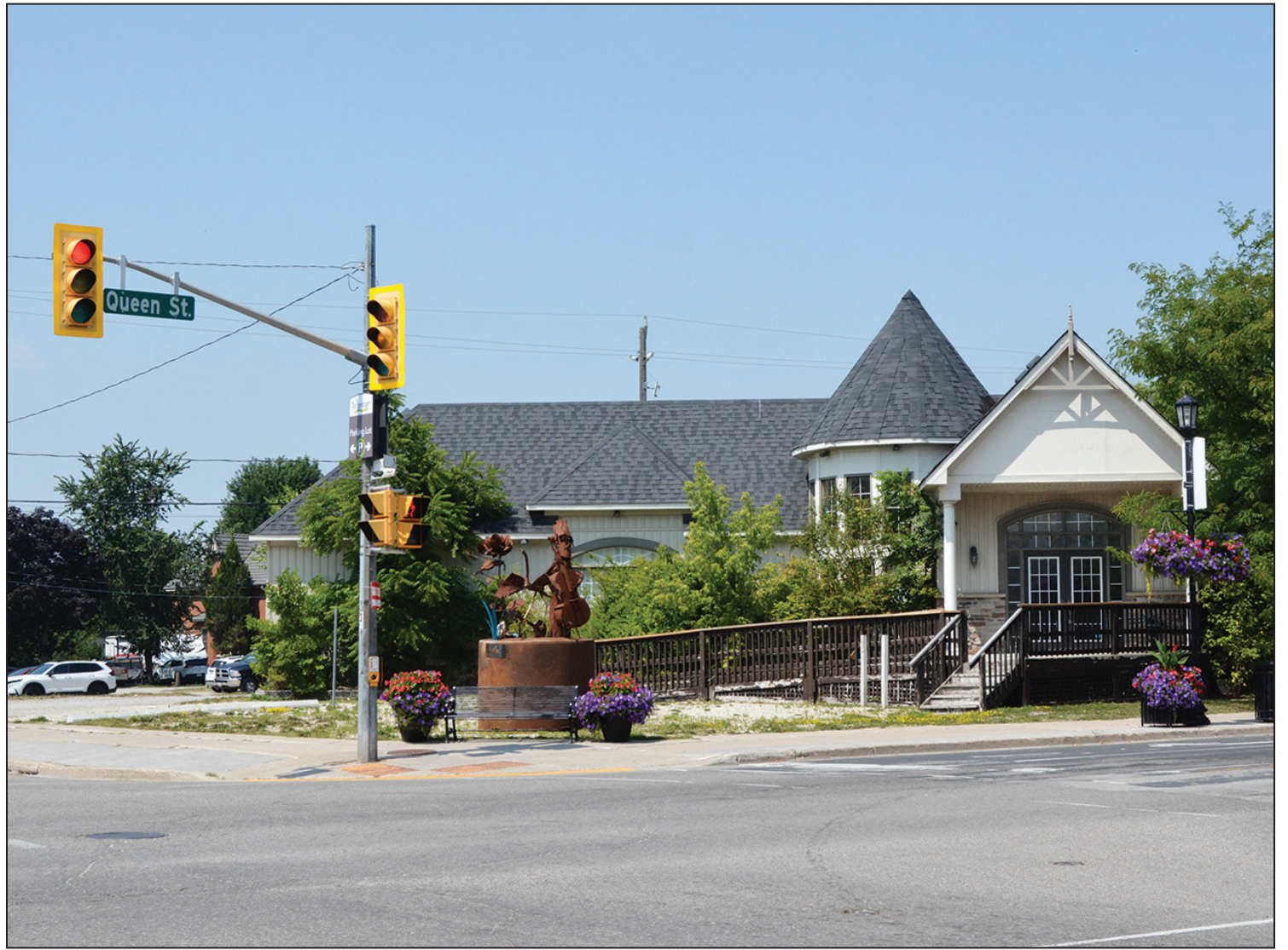
DEMO SITE – Downtown Tottenham will look a little different once demolition work is completed at the corner of Queen Street and Mill Street. The buildings are being demolished to create a parking lot. BRIAN LOCKHART PHOTO
